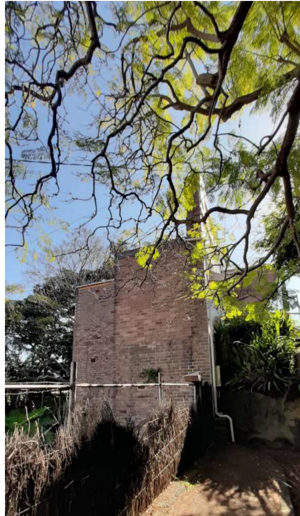
Existing East wall showing change in surrounding natural ground level, North to South
