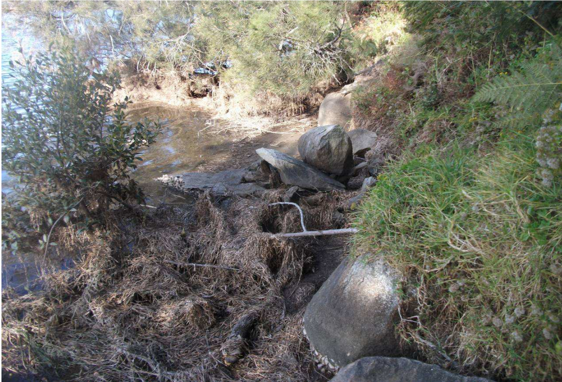
Photo 6: Granite boulders as bank stabilization immediately adjacent to the Moruya Hospital.
