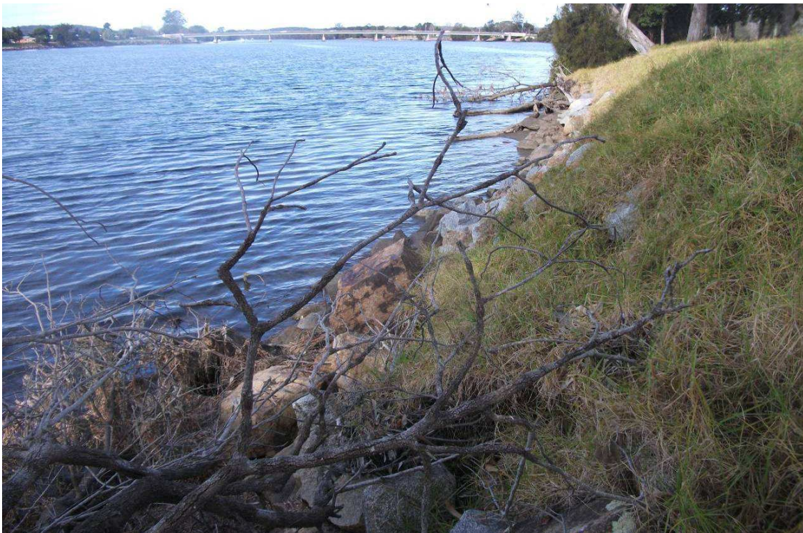
Photo 7: Granite boulders have been used for bank stabilization along most of the tidal sections of the Moruya River including between the hospital and the town centre.
